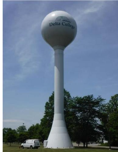
Located on Delta's Main Campus, the Water Tower is in good condition. The tank has a capacity of 200,000 gallons w/maximum diameter of 37' 11" and 135' height. Square feet based on area of water sphere at the maximum diameter. In 2010 the interior and exterior were repainted, and new safety railings and cathodic protection system were installed. In 2019 an interior leak was repaired.
