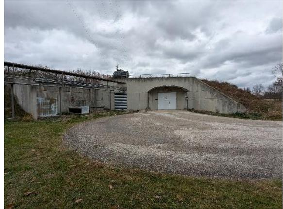
Located on Delta's Main Campus, the Radio Transmitter building is bermed on 3 sides with soil over the rooftop and in good condition. It currently is only used for analog feed of Delta College Public Media radio programming to WCMU. The rest of the area is used for storage.
