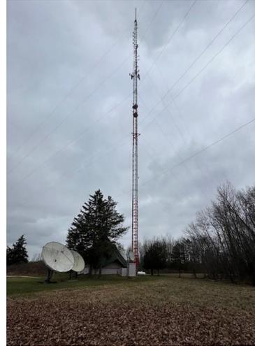
Located on the Main Campus, the TV Tower supports apertures necessary for WUCX-FM, WDCQ-TV, WTRK-FM, WLKB-FM, WSGW-FM, and Verizon Wireless. We have had several things done for the tower, including: replacing bent horizontal and diagonal bracing, plumb and tension guy wires, fix chipped concrete around base and guy anchors, replacement of lighting side markers to LED, and the most notable; the tower repainted to meet FCC/FAA regulations.
